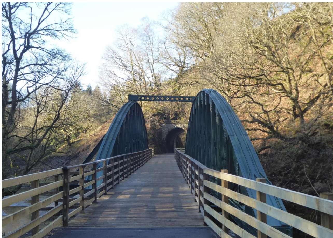
Figure 6: Keswick to Threlkeld Railway Path
